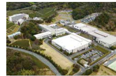
Hamamatsu Plant (Japan)
