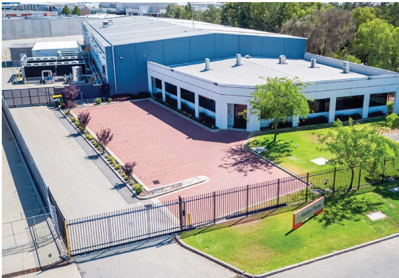
The Tier III Data Centre in Canning Vale industrial area, Perth, Western Australia
