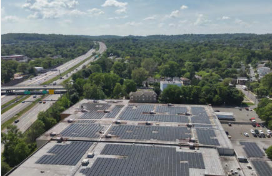
Solar Panels on the Rooftop of Millburn Self-Storage
