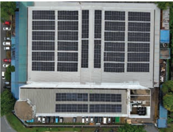
FHM - Solar panels
