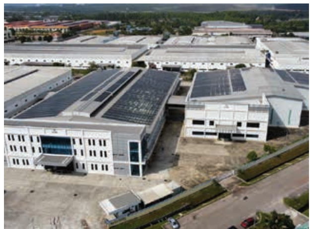
CA - Solar panels
