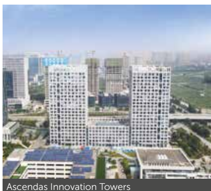
Ascendas Innovation Towers
