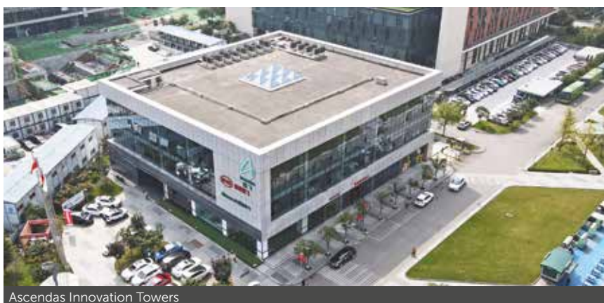
Ascendas Innovation Towers
