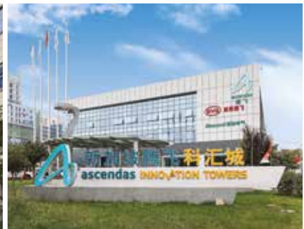
Ascendas Innovation Towers
