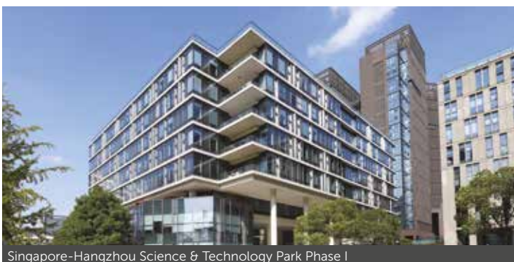
Singapore-Hangzhou Science & Technology Park Phase I
