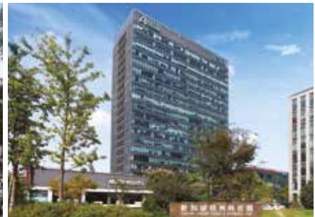
Singapore-Hangzhou Science & Technology Park Phase I
