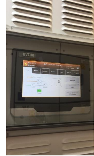
Testing of electrical system and energising the Uninterruptable Power Supply, which supplies all safety and emergency systems
