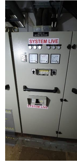
Testing of electrical system and energising the Uninterruptable Power Supply, which supplies all safety and emergency systems
