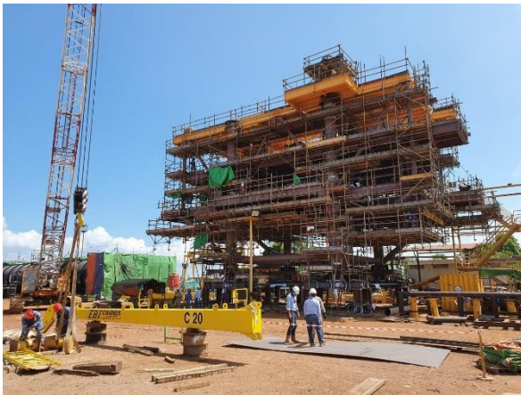
Left: Three stacked decks of Apsara platform topsides with a width of 25.4 metres at the widest point and a structural weight of 210 MT
