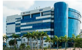
10 Changi South Lane
