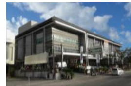
Siloam Hospitals Bali
