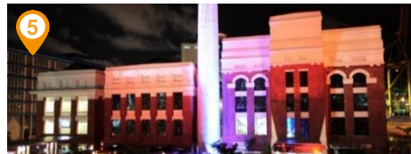
St James Power Station NLA: 119,000 sq ft
