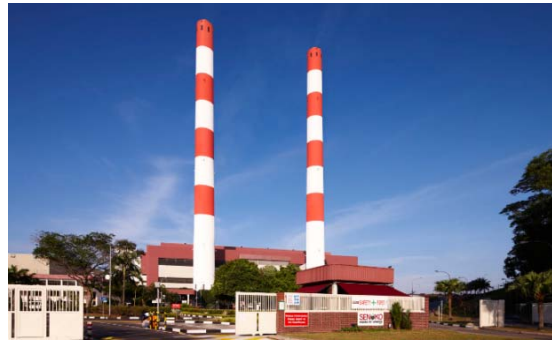
Senoko WTE Plant, Singapore
