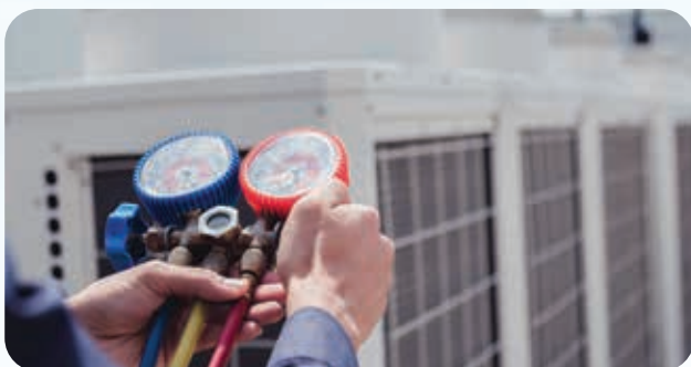
Commercial maintenance servicing in progress
