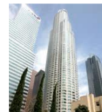
U.S. Bank Tower, Los Angeles (100% stake)
