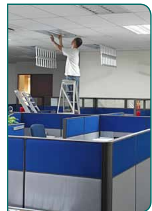
Replacing fluorescent lighting with energy-efficient LED lighting
