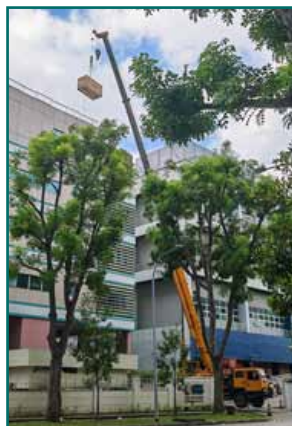
Hoisting of solar panels
