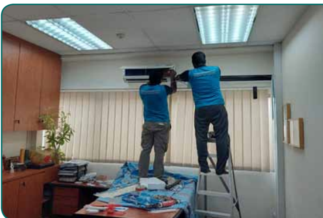
Replacing the air-cons with energy efficiency 5x green ticks mark
