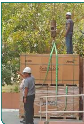
Hoisting of solar panels
