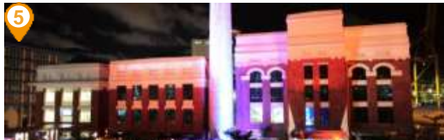
St James Power Station NLA: 66,000 sq ft
