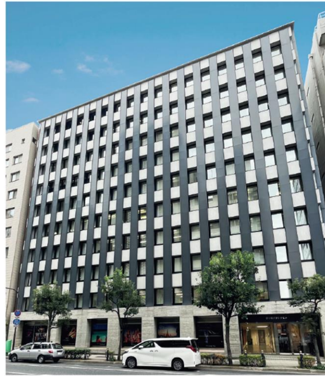
YOTSUBASHI GRAND BUILDING, BROAD STREET FRONTAGE ON YOTSUBASHI SUJI, SHINSAIBASHI • LAND AREA - 881 SQM • GFA - 7,524 SQM • EFFECTIVE OWNERSHIP - 53%
