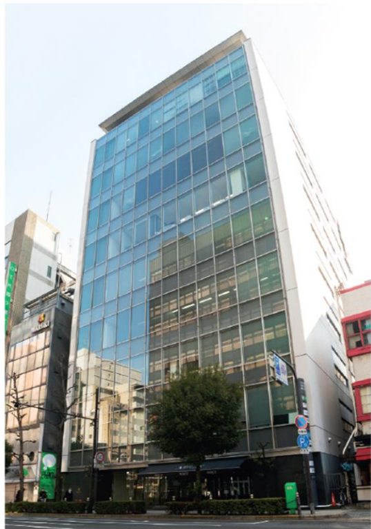
YOTSUBASHI NAKANO BUILDING ALONG YOTUSBASHI SUJI, SHINSAIBASHI • LAND AREA - 806 SQM • GFA - 7,925 SQM • EFFECTIVE OWNERSHIP - 50%
