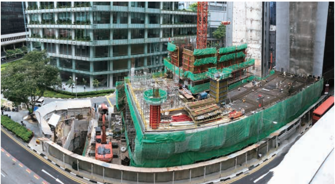
Robinson Tower Redevelopment – on track to its completion in 2018.
