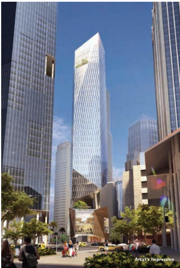
Robinson Tower Redevelopment – less than 100 metres from Raffles Place MRT.
