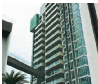
Sennett Residence, Singapore
