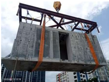
Securing webbing sling around the PPVC as an additional measure.
