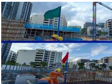
Using green and red flags to indicate safe and unsafe work zones.
