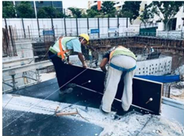
Using self-retracting lifelines when working near unprotected edges.
