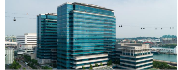
Keppel Bay Tower is Singapore's first commercial building to be fully powered by renewable energy and certified BCA Green Mark Platinum (Zero Energy)
