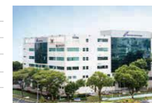
30 Marsiling Industrial Estate Road 8
