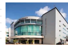
25 Changi South Ave 2
