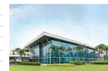
3 Tuas South Ave 4
