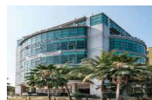
2 Tuas South Ave 2
