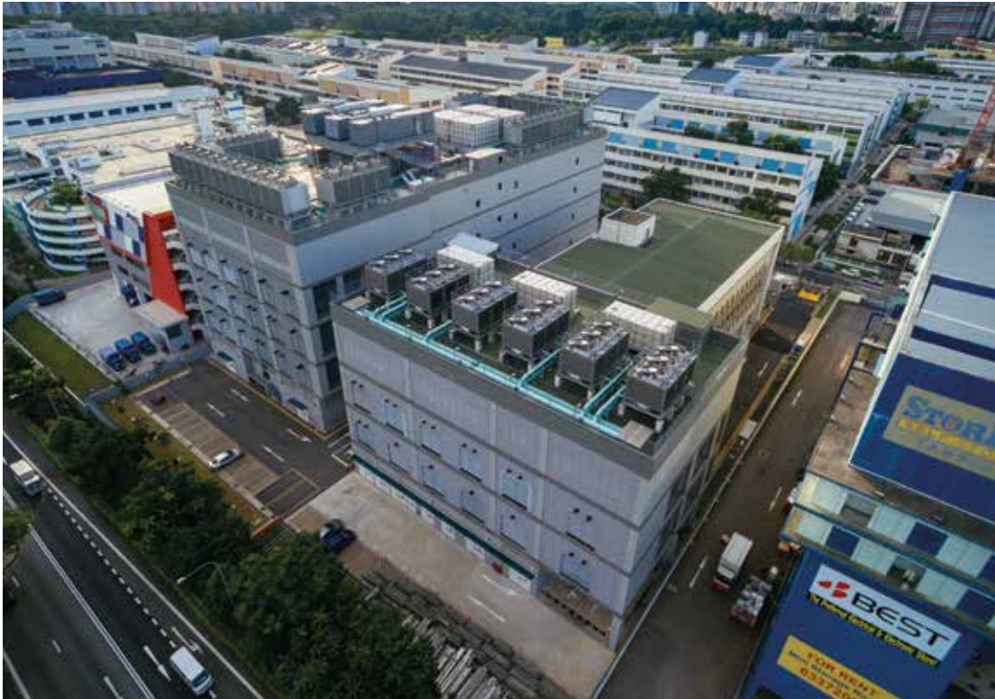
Increasing the cooling tower water recycling capabilities at KDC SGP 1 and KDC SGP 2 reaped water usage intensity improvements.
