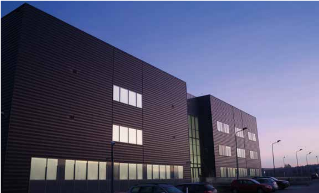
Amsterdam is one of five main data centre hubs in Europe.
