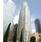
U.S. Bank Tower, Los Angeles (100% stake)
