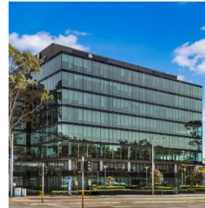
Dec 2020: Acquired Pinnacle Office Park in Sydney
