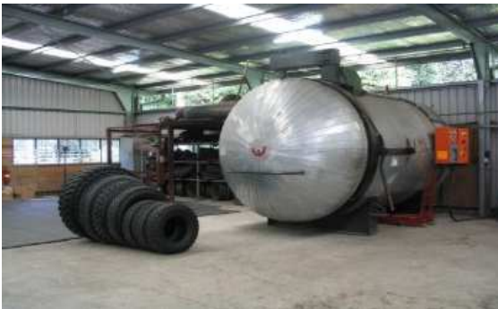
Tyre retreading plant, Timika
