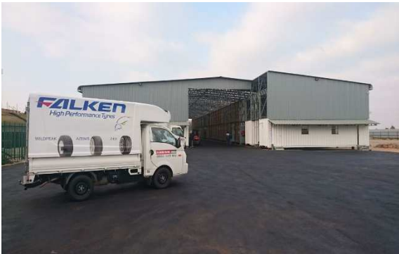
New container warehouse in Johannesburg, South Africa
