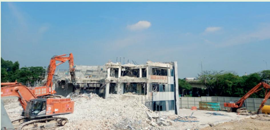
98% of construction materials were recycled during the demolition at 51 Benoi Road in Singapore
