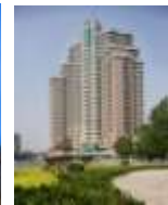
Somerset Olympic Tower Property Tianjin
