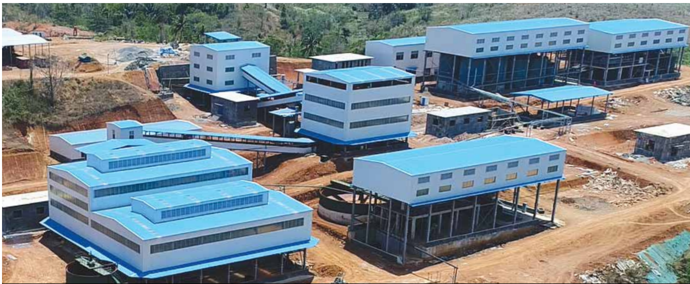
Tampilan keseluruhan dari fasilitas pengolahan floatation and carbon-in-leach berkapasitas 500 ton per hari Overall view of the 500 tonnes per day floatation and carbon-in-leach processing plant
