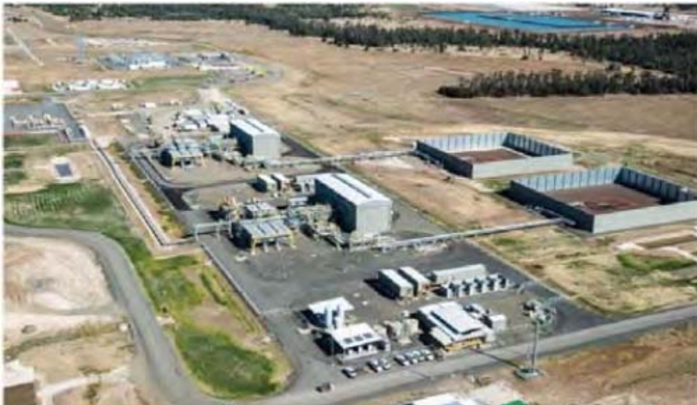
Condabri Central Gas Processing Facility
