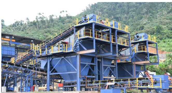
Plant and machinery deployed at the Chaah Mine
