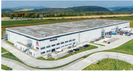
1 Nove Mesto ONE Industrial Park I, Beckov
