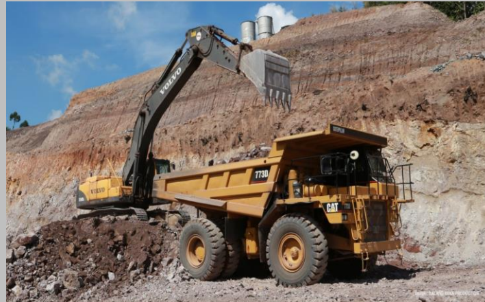
Dumper and excavator
