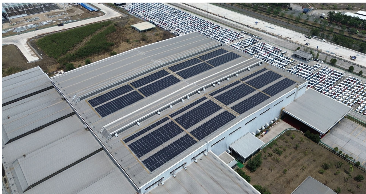
Solar panels at PT Astra Daihatsu Motor
