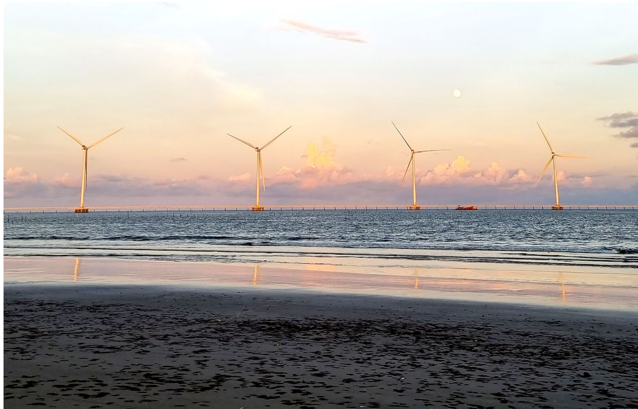
REE's Tra Vinh V1-3 Wind Power Plant
