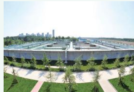
Shandong Ji'nan Waste Water Treatment Project
