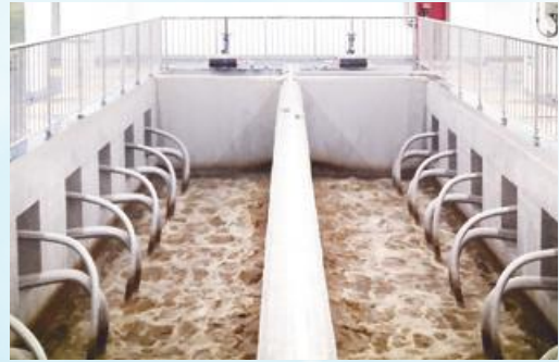
Ji'nan Huashan Waste Water Treatment Project 濟南華山水質淨化項目
