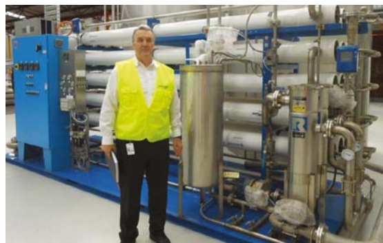
Reverse Osmosis (On-site Water Recycling Plant)
