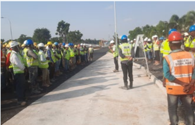
Toolbox meeting being held at OKP's construction site.
