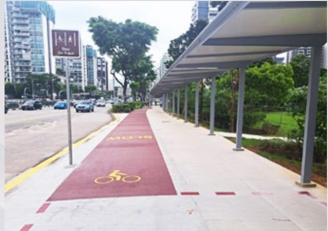
Completed work using CMC at new Cycling Path Network project at Potong Pasir town.
