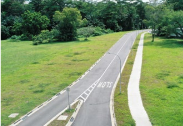
New access road at Loyang Valley for OKP's project involving commuter and road infrastructure works in Pasir Ris and Loyang.
