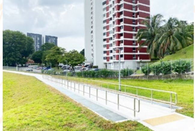
One of OKP's ongoing projects is road maintenance contract for South East Sector.
