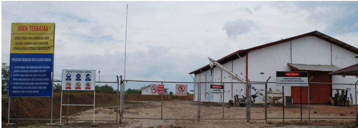
Figure 4.21 – Explosive Magazine Completed
