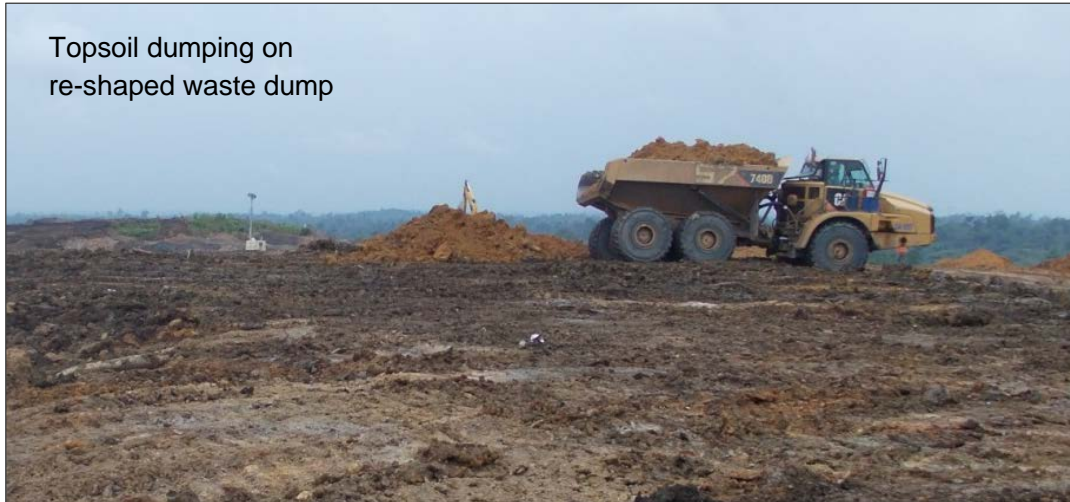
Figure 5.4 – Topsoil Handling and Rehabilitation
