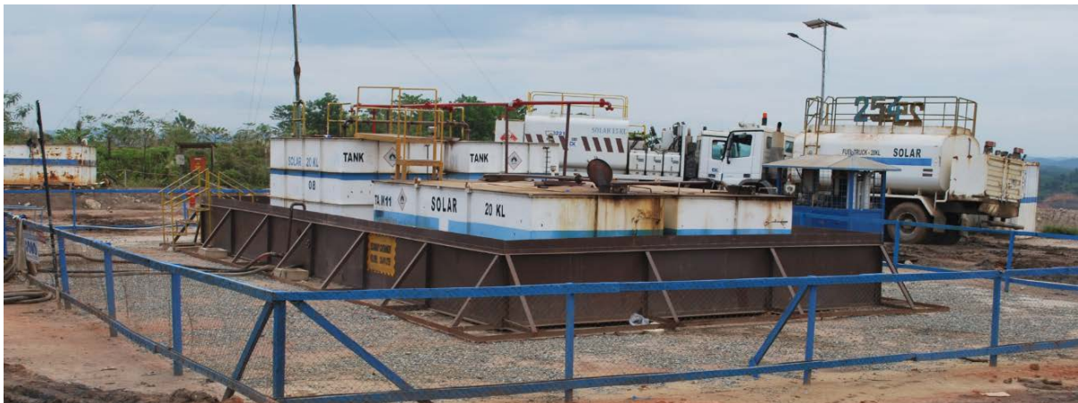
Figure 4.19 - Fuel Storage and Distribution Facility Completed
