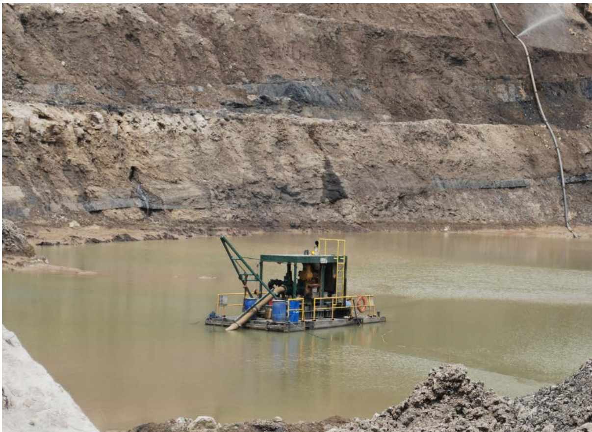
Figure 4.14 – Pioneer 90 Litre per Second Dewatering Pump
