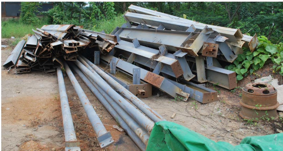
Figure 4.22 - Building Materials on Site Ready for Construction of New Workshop
