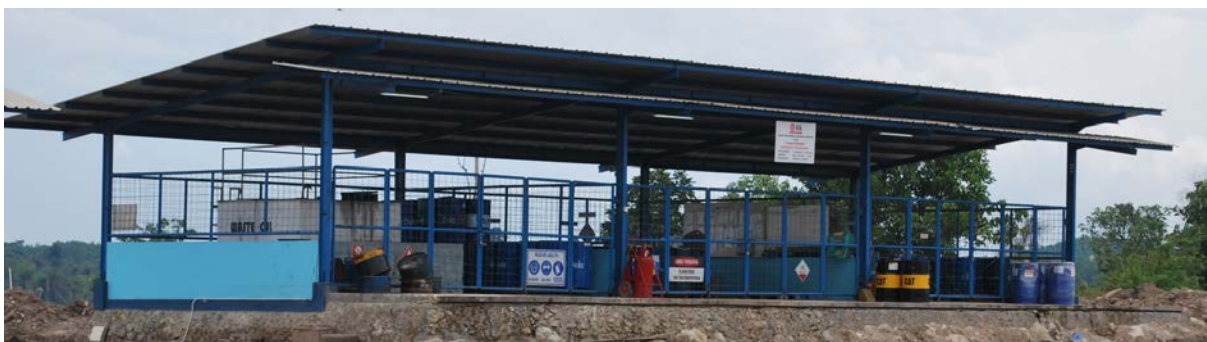
Figure 4.20 - Oil and Other Hydrocarbon Storage Facility Completed with No Bund
