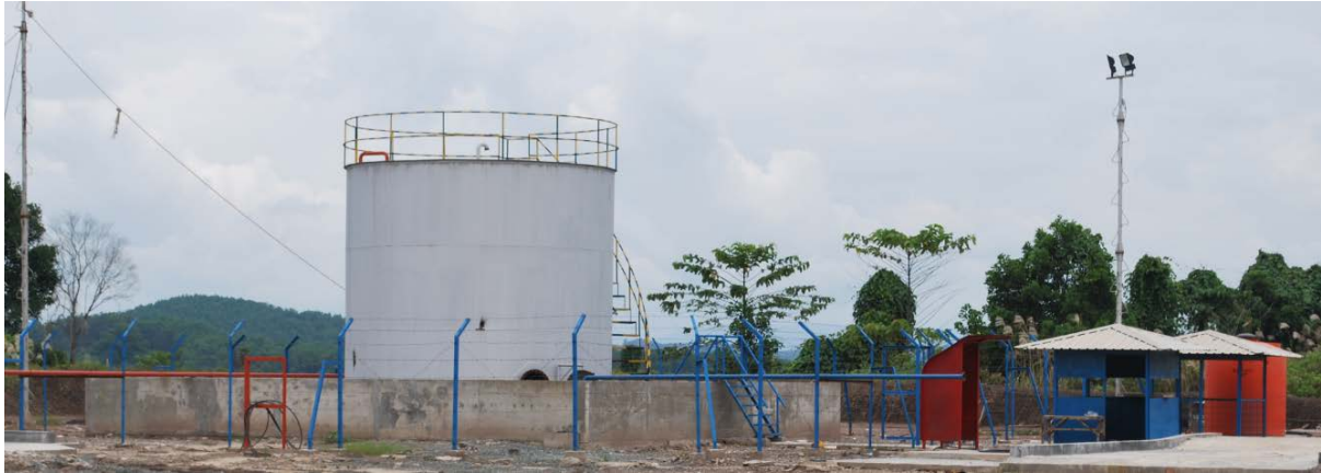
Figure 4.18 – New Fuel Storage Facility Waiting on Permit
