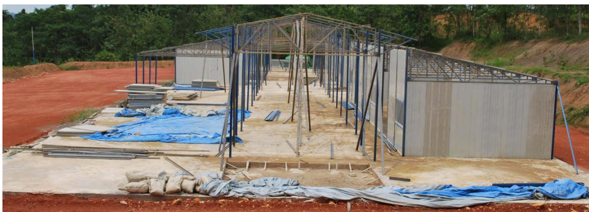
Figure 4.23 – Construction of New RK Site Office
