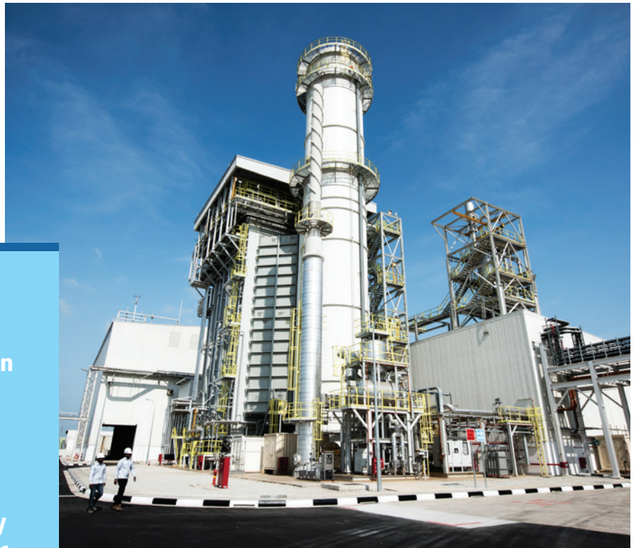
Tuaspring Power Plant, Singapore
