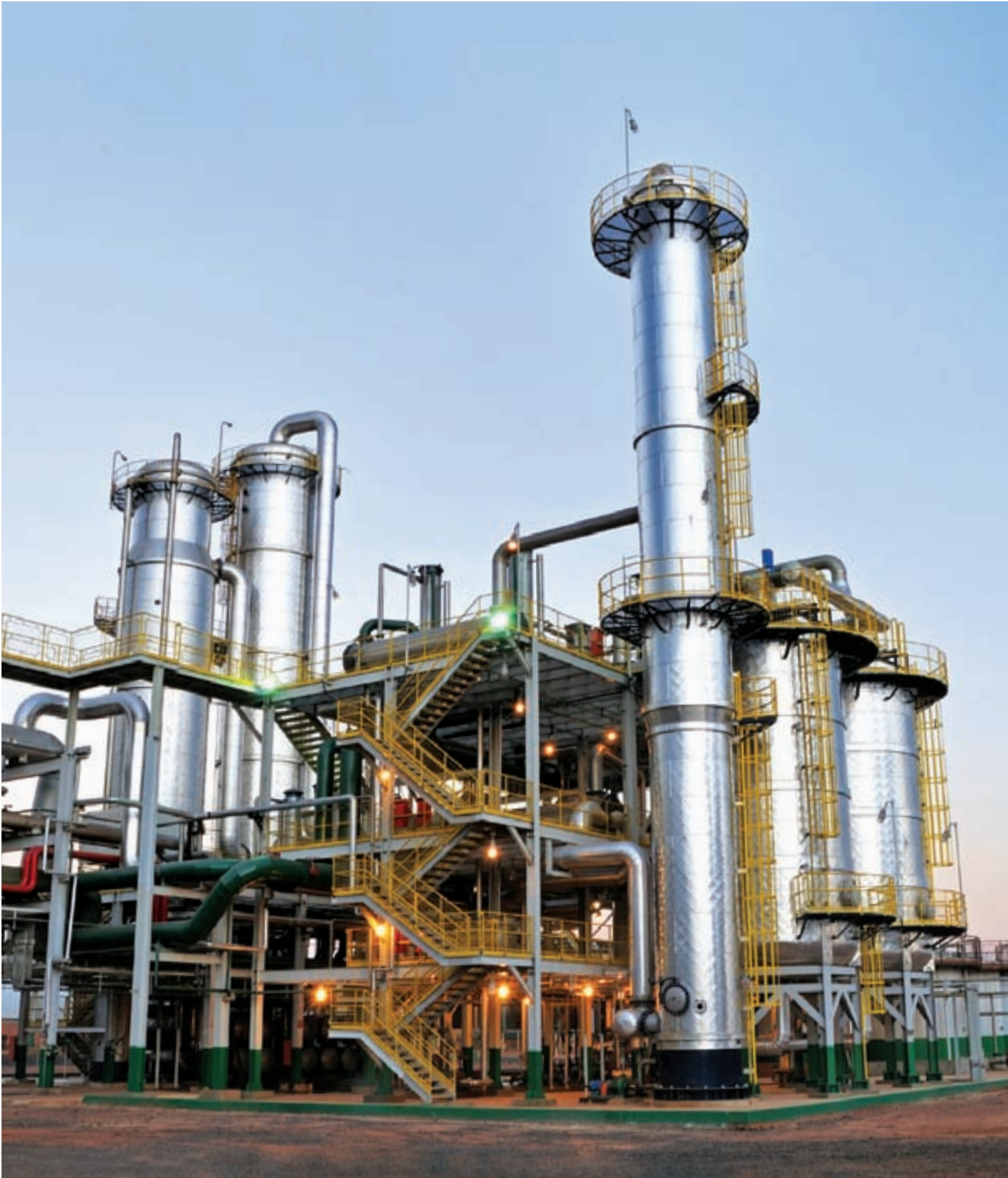
CMAA sugar mill and ethanol plant in Brazil
