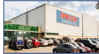
20 217 – 225 Boundary Road, Laverton North
