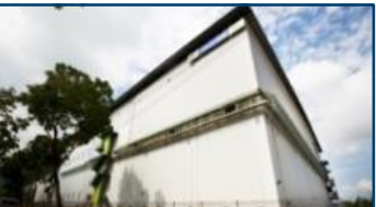
2 Cache Cold Centre 2 Fishery Port Road
