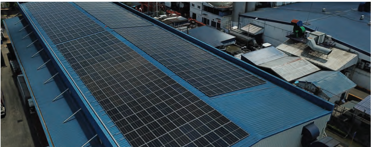
New solar panels were installed at Gardenia Philippines in FY2023.
