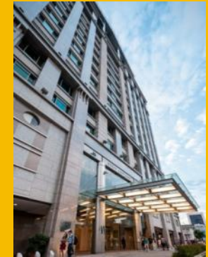
Bugis Junction Towers (100% interest)
