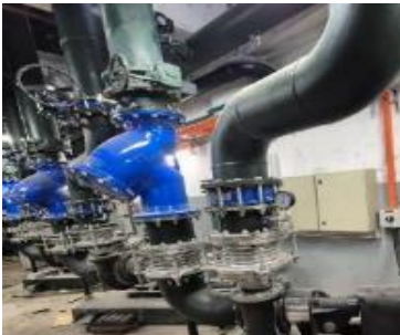
Completed chiller system replacement in Wisma Atria Property on Cooling-as-a-Service scheme
