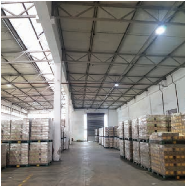
Installation of LED lights in Johor Bahru Plant
