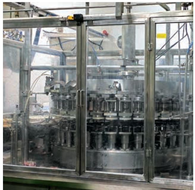
Clean-In-Place System in China Guangzhou Plant
