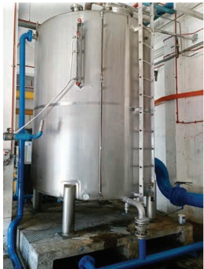
New Condensate Recovery System in Shah Alam Plant
