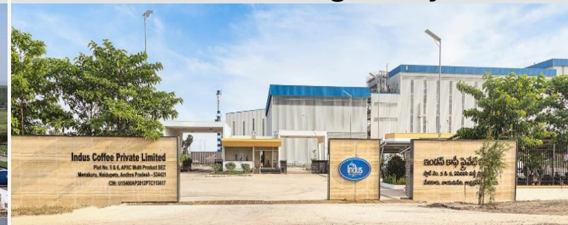
Freeze-dried soluble coffee manufacturing facility
