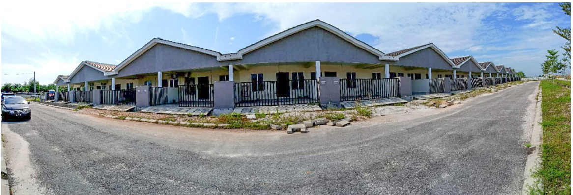
Sri Iskandar's terrace houses in progress
