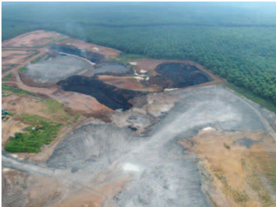
Figure 9:2 Current Mining at SN Pit
