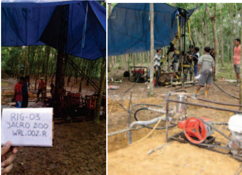
Figure 4:3 WRL Drilling Operations
