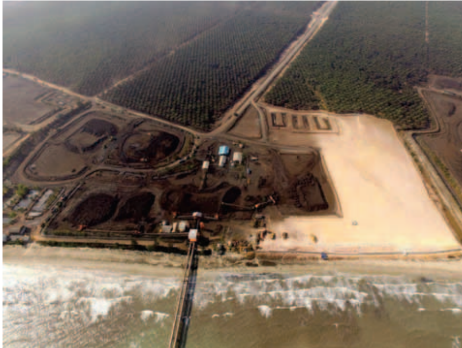
Figure 9:5 Coal Loading Facilities at Port
