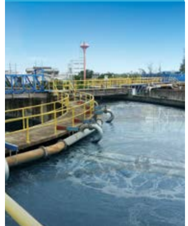
Bang Poo Waste Water Treatment Plant
