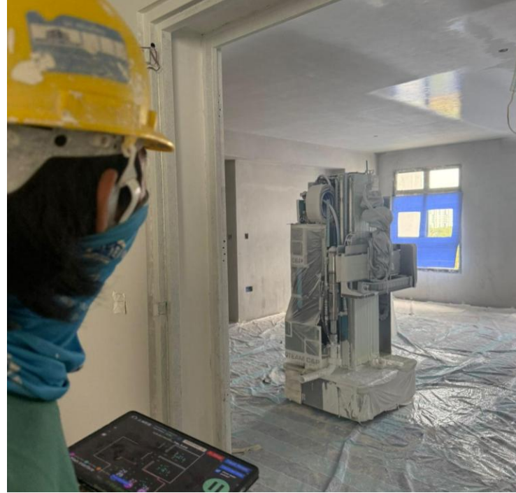
C&P: Indoor Painting Robot @ HDB flats at Tengah C8
