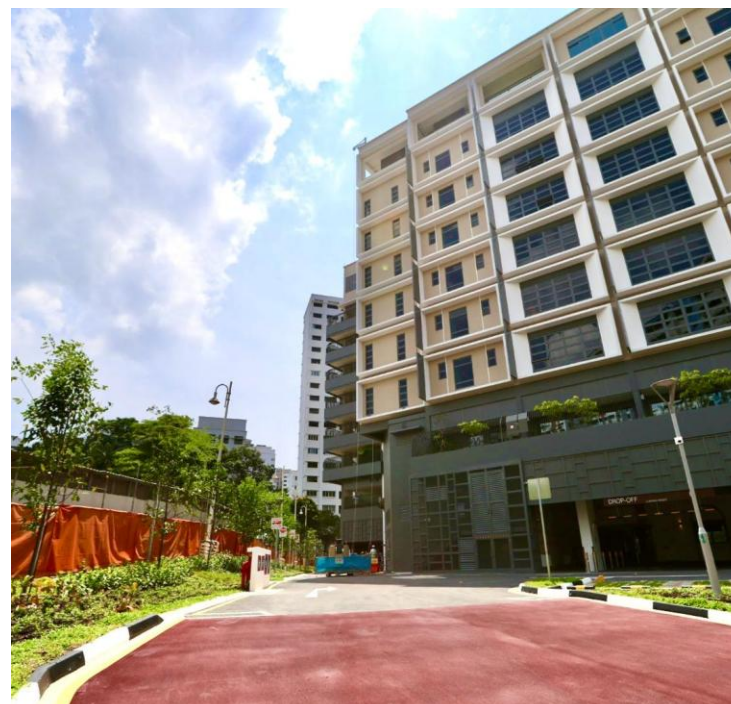
Saint Luke Hospital
