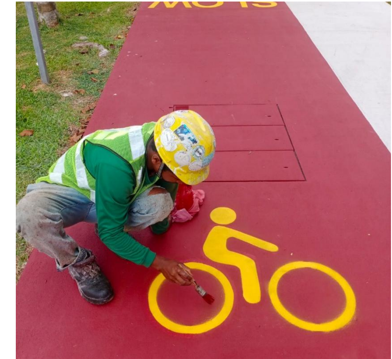
Epoxy flooring @ Cycling path
