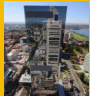
Old Treasury Building Office Tower, Perth (50% interest)
