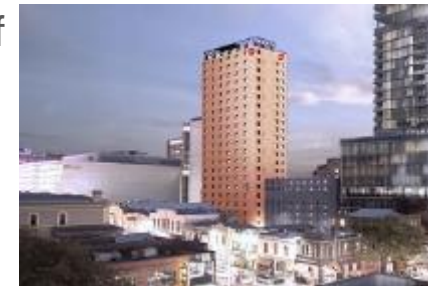
dwell Adelaide • 280 beds • Land tenure: Freehold • Land area: 598 sqm • Located close to University of Adelaide and University of South Australia – City East Campus • Development completed in Oct 2018, and began accepting occupancy in Jan 2019
