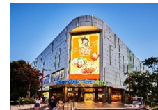
Northpoint City North Wing 2017
